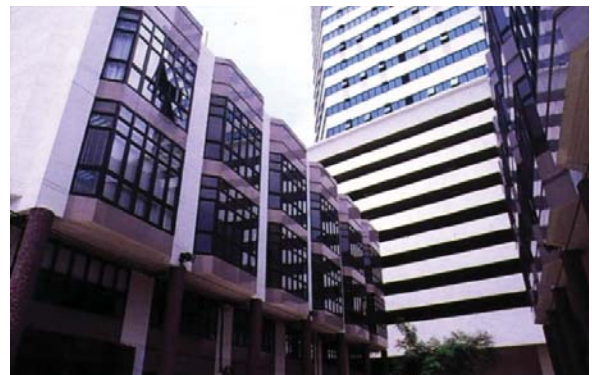
Vongvanij (Building C), V International Property Co.,Ltd Scope of service : Design + CM Year : 1994 - 1998
