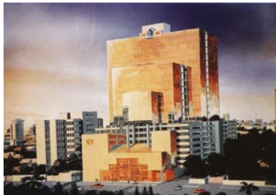
Richmond Office, Shining Condo Co.,Ltd Scope of service : Design + CM Year : 1990 - 1992
