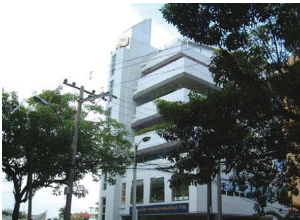
BECTHAI Head Office, BECTHAI Bangkok Equipment & Chemical Co.,Ltd Scope of service : Design Year : 1998
